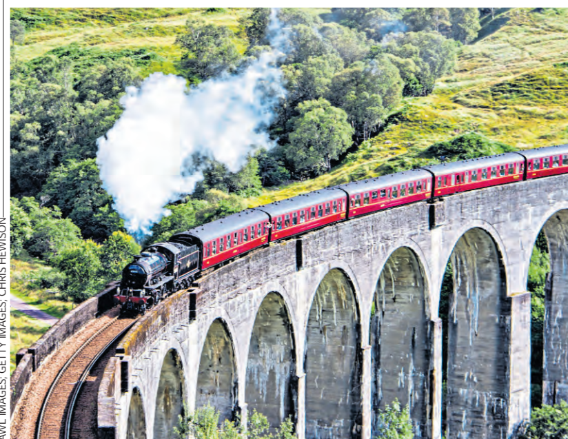
TAKE THE HIGH ROAD The Jacobite crosses the Glenfinnan Viaduct, Scotland
